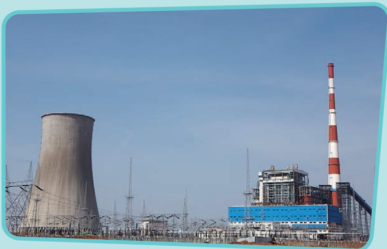
Kakatiya Thermal Power Plant 1x500 MW BoP APGENCO, Warangal Andhra Pradesh | June 2010
