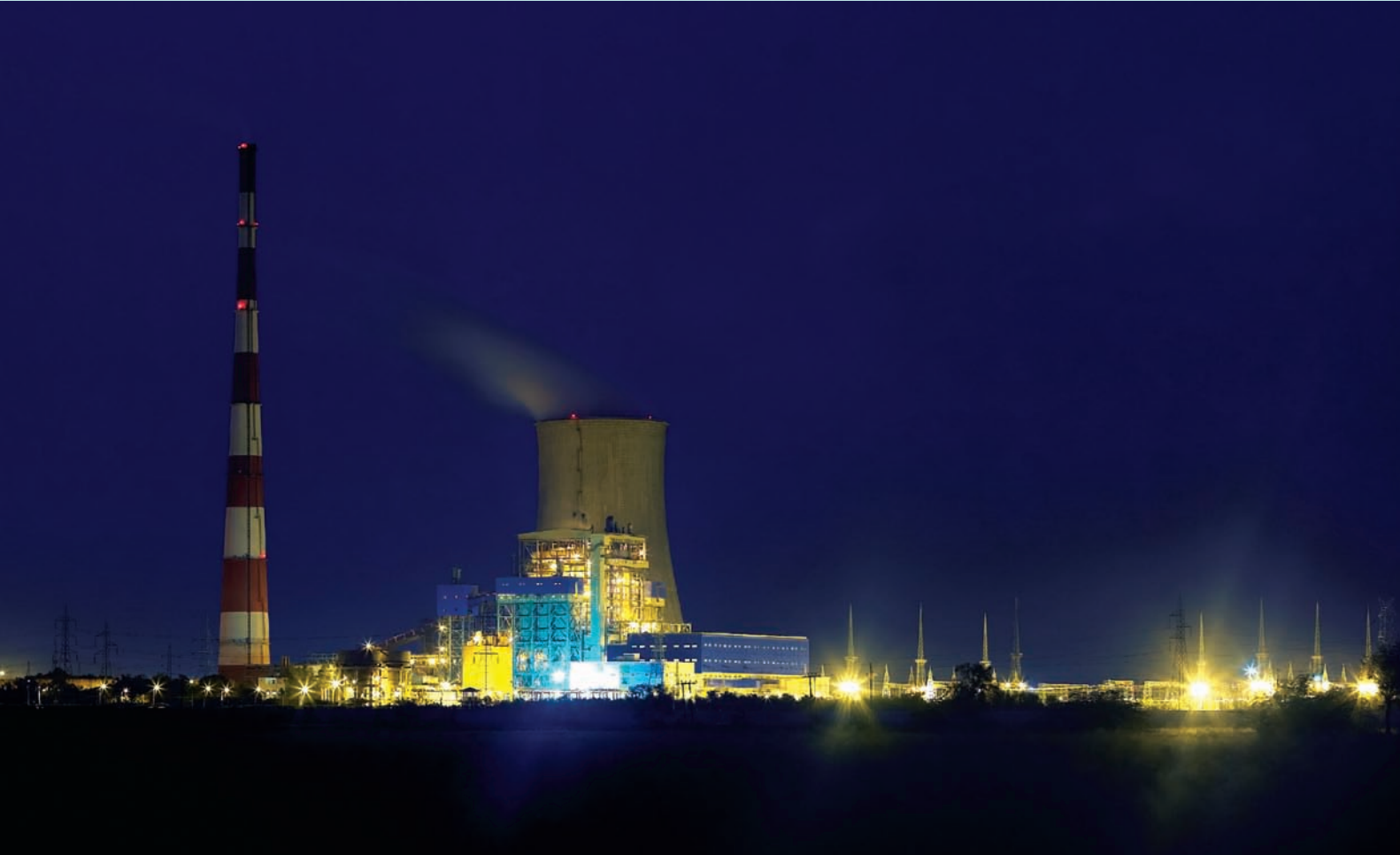
500 MW Vijayawada Thermal Power Station Stage - IV, APGENCO, Andhra Pradesh
